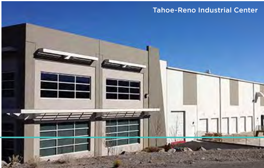
Tahoe-Reno Industrial Center
